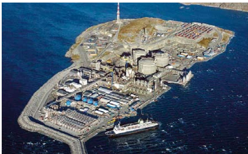
A priority in the Barents Sea is finding sufficient quantities of gas in the area around Snøhvit to justify a second process train at the Melkøya gas liquefaction plant.
