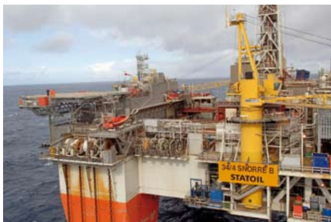
The Tampen region of the northern North Sea is an example of area development based on existing fields, such as Snorre.
